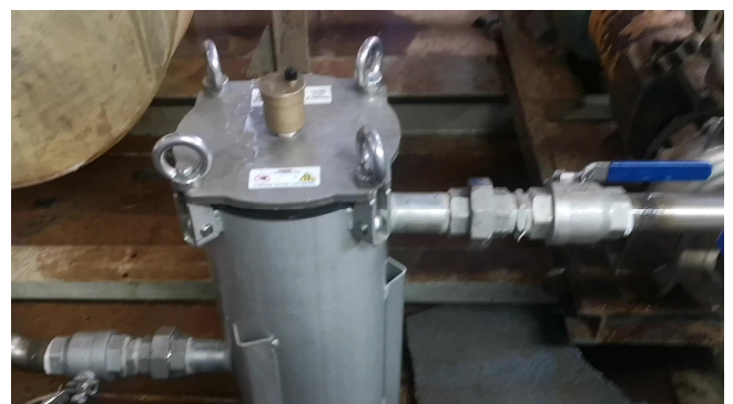
Magnetic filter installation.
